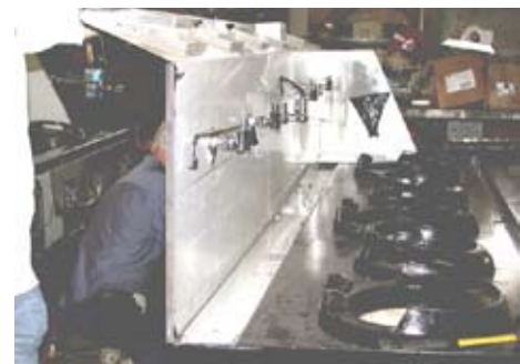
8. When raised, the gutter and backsplash should be aligned. Bolt side splashes to body.
